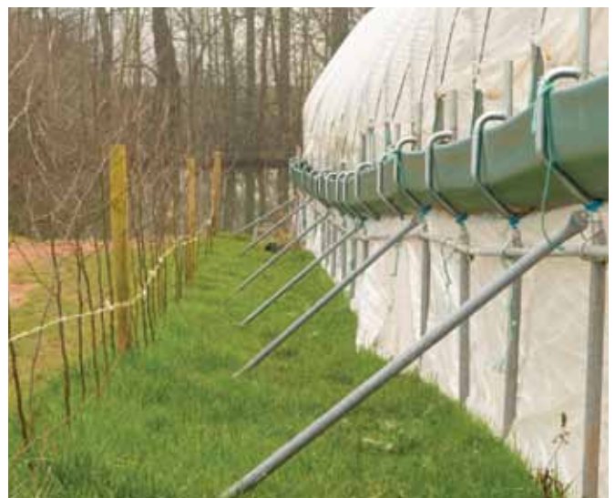
Harvested rainwater is collected from polytunnels in the guttering shown and then collected in the lined reservoir to be used for irrigation
