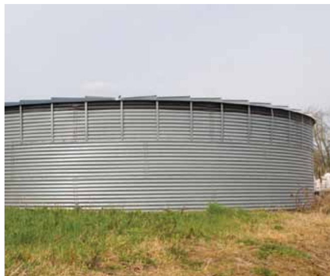
A new large above ground store
