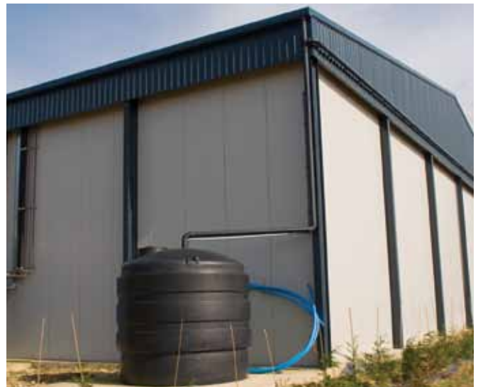
The amount of rainfall that can be collected depends on your roof area
