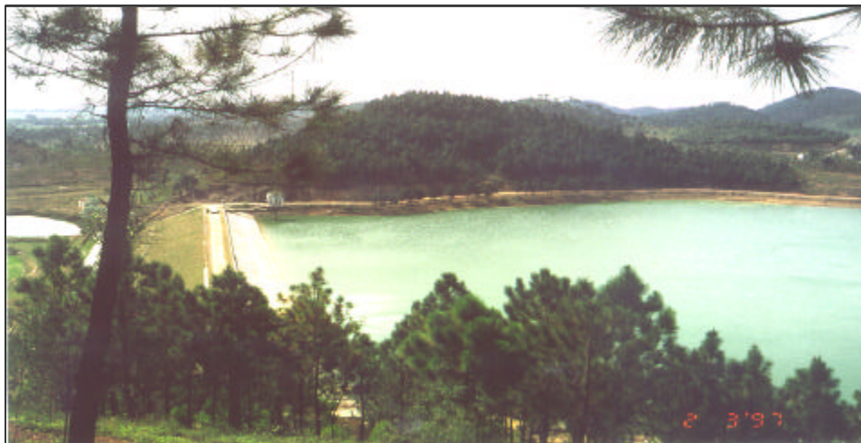
Figure 6 : Rainwater reservoir in Northern Vietnam (1.300 mm/a rainfall); water being used for paddy cultivation
