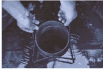
5. Take out the locking device and lift it out of the shaft
